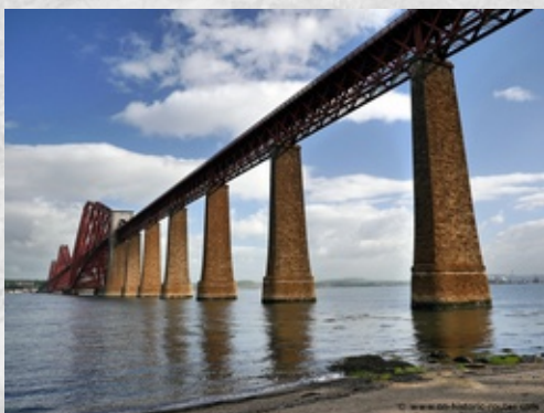
Rail bridge across the Firth of Forth near Edinburgh.
